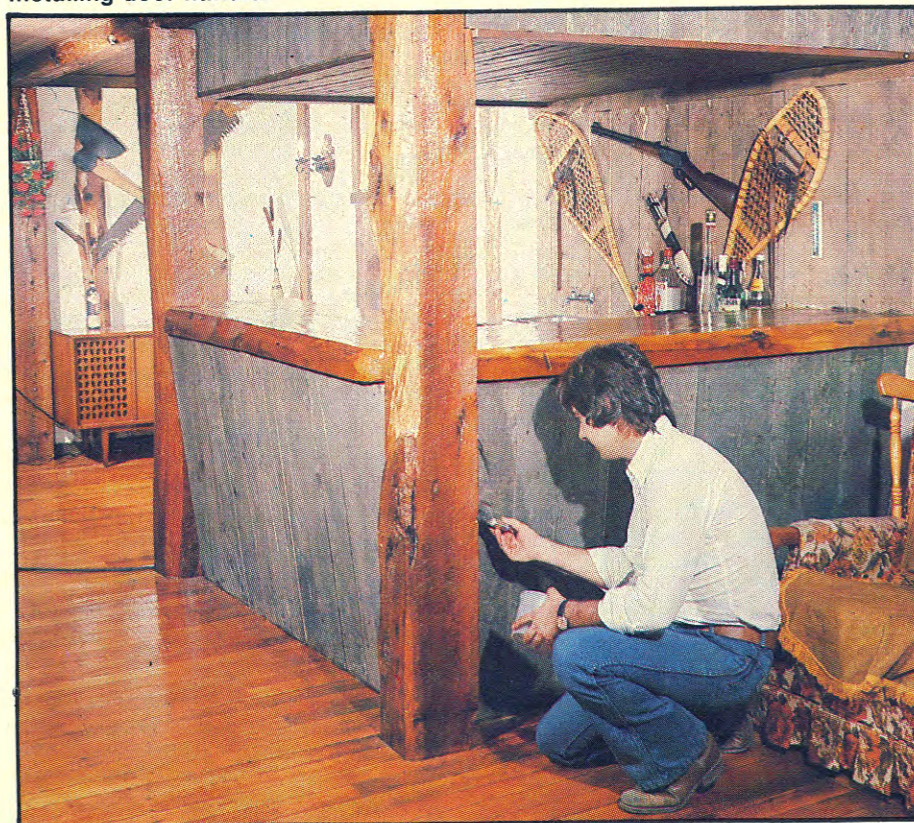
Finishing countertop and beams with a plastic finish.
